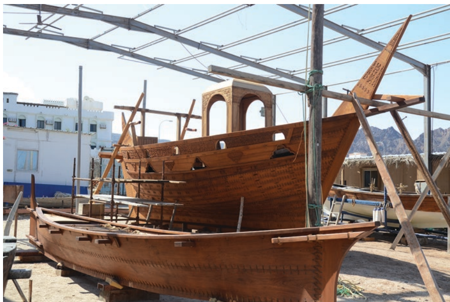
Fig. 8.3 The al-Hariri Boat and the beden seyad under construction in the Oman Maritime boat-yard. (Photo courtesy of the author)
